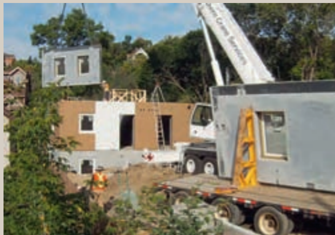
Construction of an innovative duplex residence designed to achieve zero net energy use. The use of pre-cast concrete panels, produced at a nearby Lafarge facility, allowed for fast and efficient on-site assembly.
